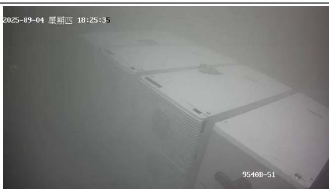
Figure 2.24: During 3 rd cell (cell 6) venting (Local Time in 18:25)
