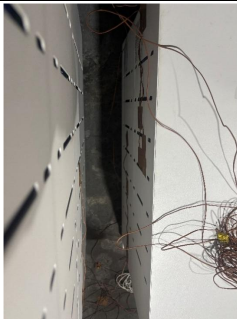
Figure 2.16: Thermocouples on Column A
