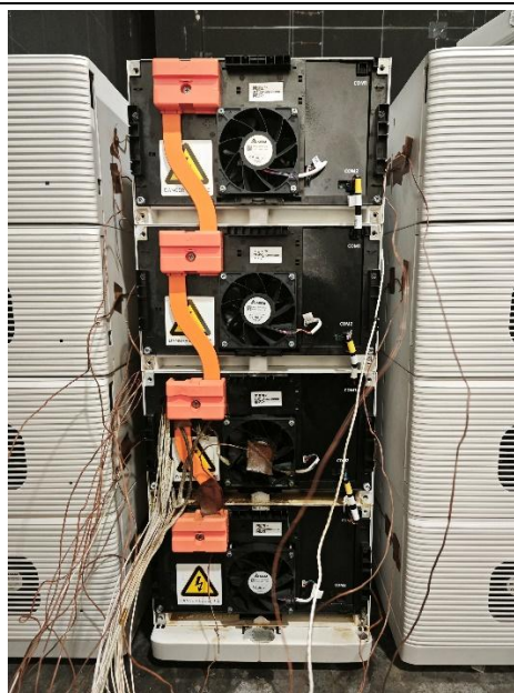
Figure 2.46: Front view of Column B after test
