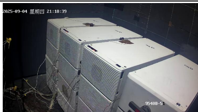
Figure 2.34: During cell 10 venting (Local Time in 21:18)
