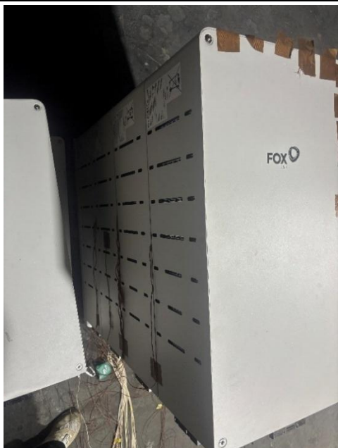
Figure 2.15: Thermocouples on Column B
